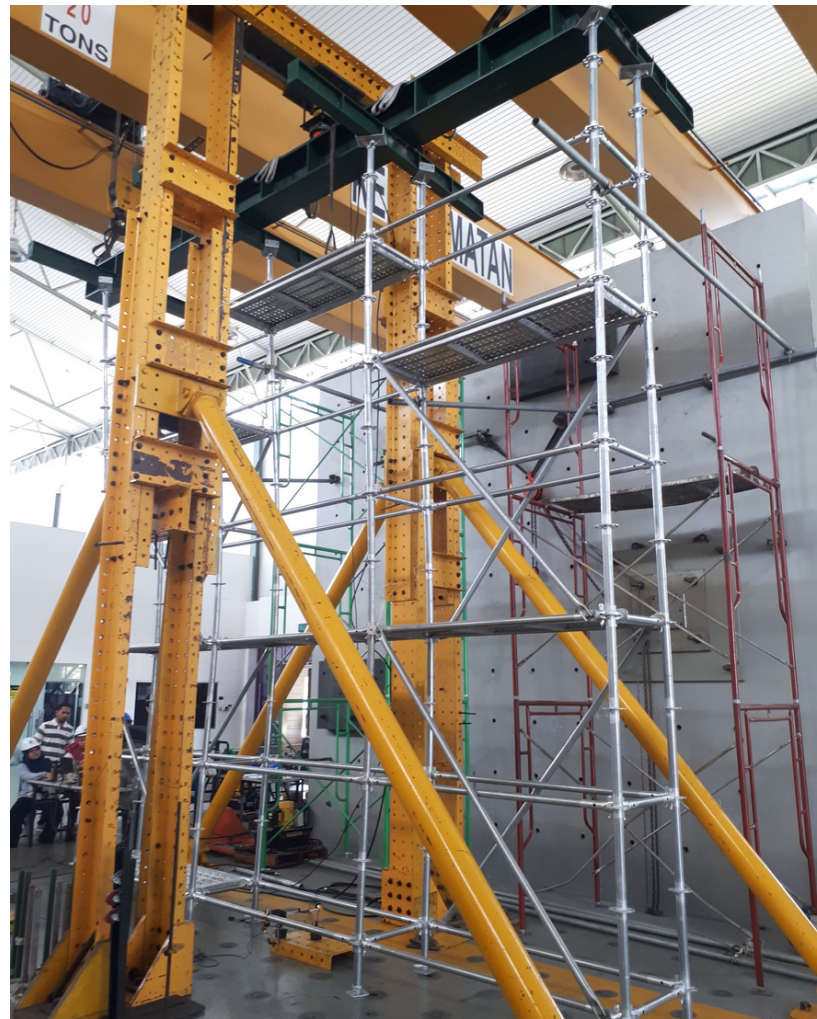
Full load tower test on falseworks
